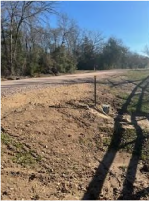
Figure 12 – Dove Lane Culvert Replacement and Base Installation 1/13/2026
