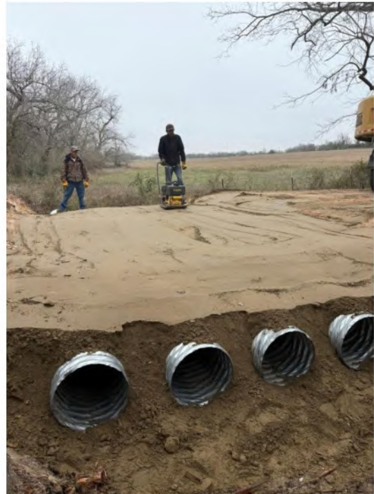
Figure 21 – Culvert Backfill Compaction (Cement Stabilized Sand) 1/22/2026
