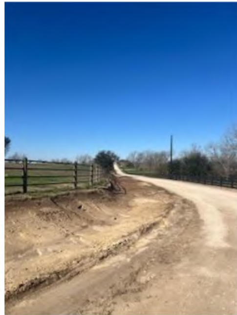
Figure 11 – Egypt Road Ditching and Road Widening 3/3/2026
