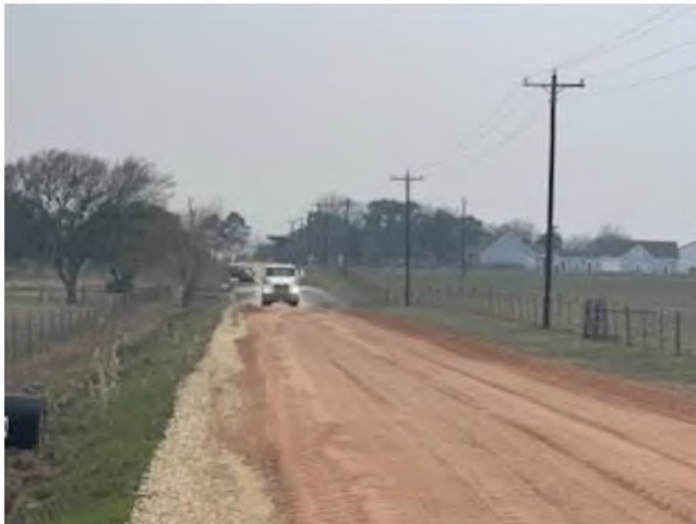
Figure 13 – Maass Road Base Installation 2/19/2026
