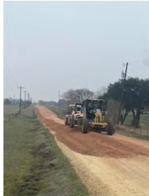
Figure 14 – Zibilski Road Base Installation 2/23/2026
