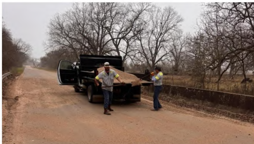
Figure 23 - Winter Storm Fern Bridge Deicing 1/23/2026
