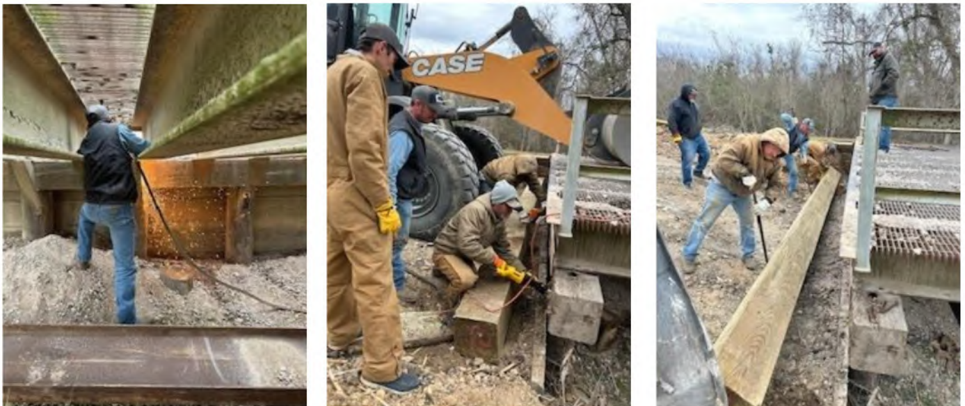
Figure 18 – Deer Point Road Bridge End Cap Replacement 12/29/2025
