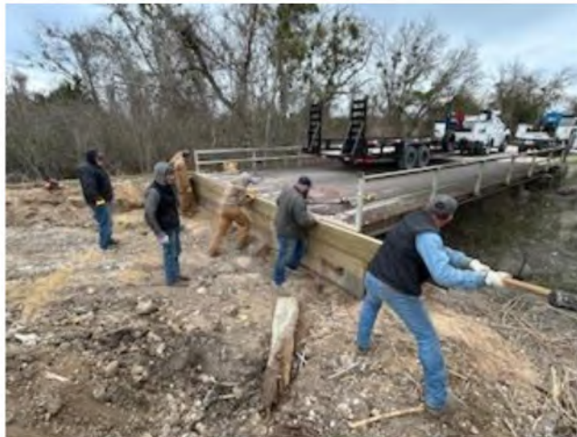
Figure 19 – Deer Point Road Head Wall Installation 12/29/2025
