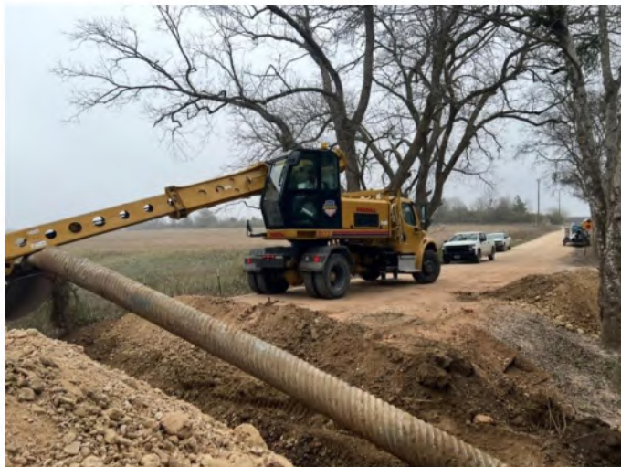
Figure 22 - Meyersville Culvert Removal 1/22/2026
