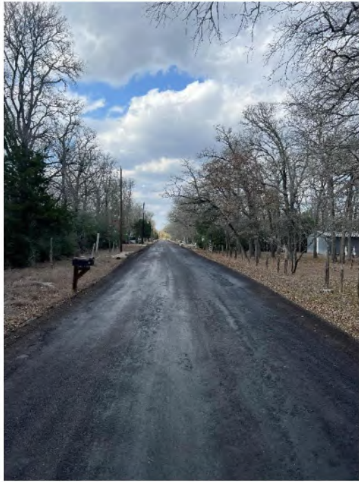
Figure 15 - Edgewater RAP Installation – 2/12/2026
